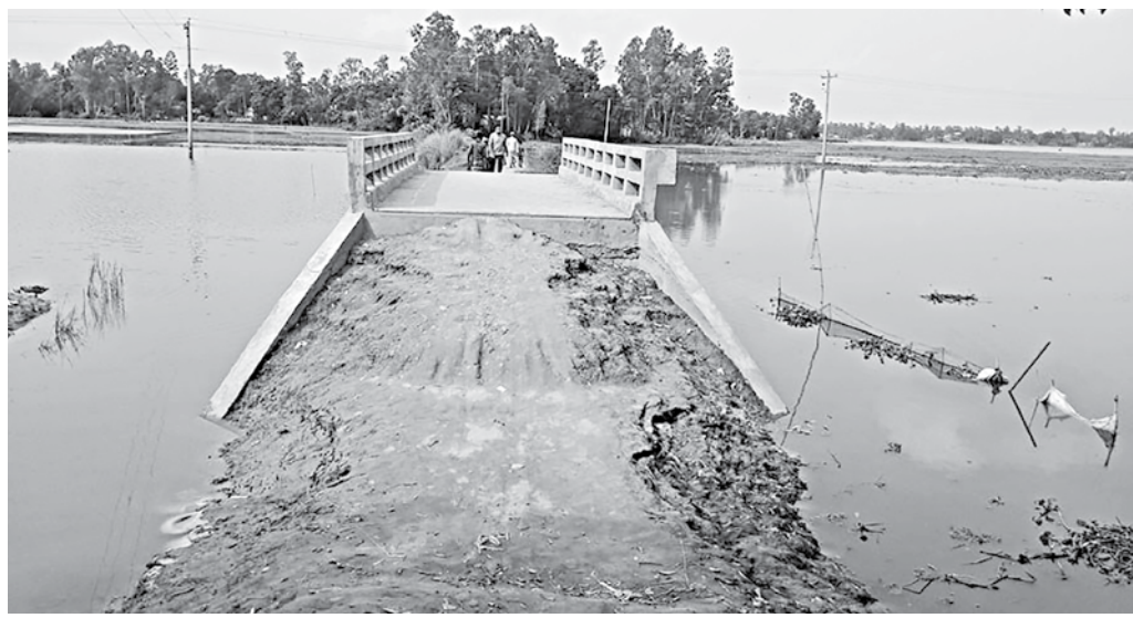
The skeleton of a road, a culvert, is what remains after floodwaters receded from Porjana village in Shahzadpur upazila of Sirajganj. The photo was taken on last Sunday. PHOTO: STAR
