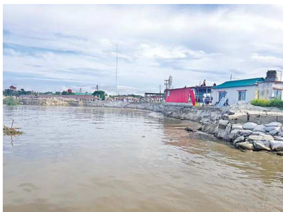
The Padma is rapidly eroding its banks near Shimulia ferry terminal in Munshiganj, devouring at least 10 acres of land in less than a day. Ferry services have completely stopped with residents scrambling to get their movable belongings to safety. The photo was taken yesterday.
