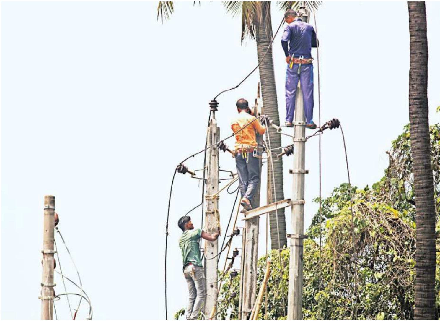
A group of Dhaka Power Distribution Company staffers were spotted yesterday fixing electrical poles at Kalyanpur, opposite the Khaleque Service Station. Though the task carries risk of fatality from electrocution, none of the workers seem to be wearing any protective gear, an issue persists despite repeated condemnations from activists and coverage in press.
