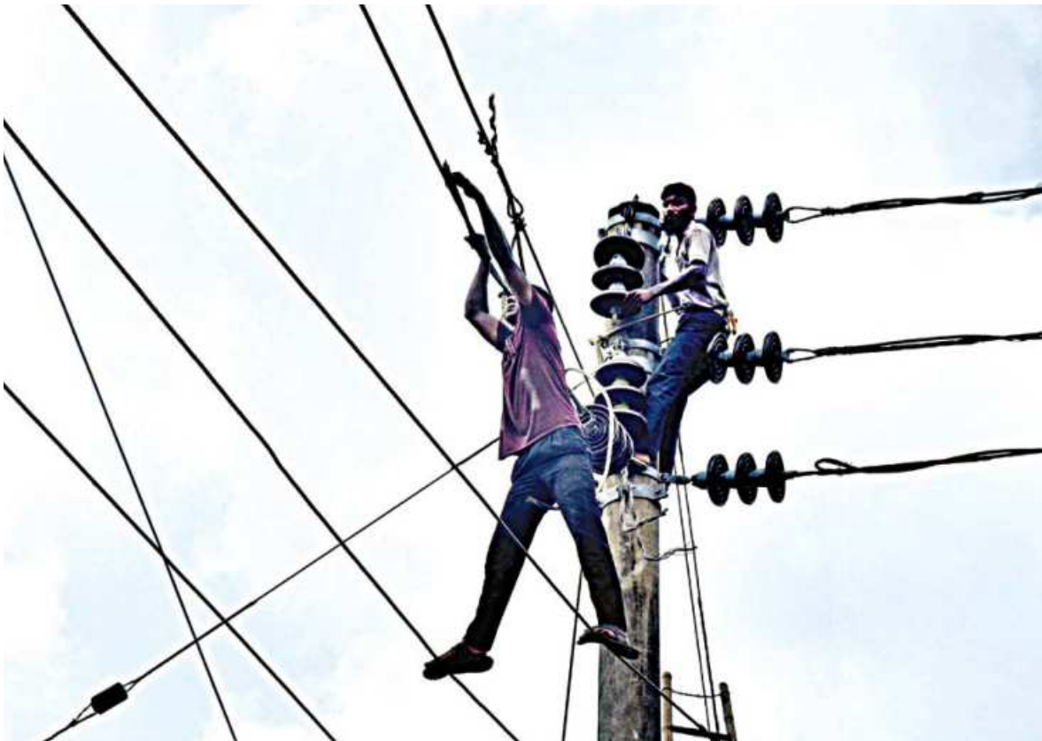
Without any sort of safety gear, two men work to repair a line from a 48-feet-high electric pole in Banda Road area of Barishal city. Such unsafe and dangerous acts go unabated due to weak enforcement of labour laws in the country. The photo was taken on Sunday.
