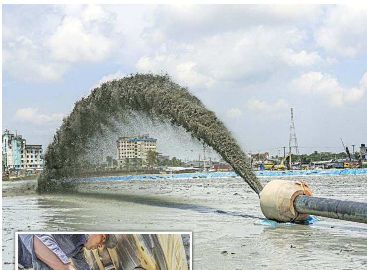
Dredging of the Karnaphuli river resumes after being suspended for a long time because of the pandemic. But the challenge is discarded plastic goods at the bottom of the river clogging the machine in about every 15 minutes. Inset, mechanics removing plastic bags from a cog yesterday.
