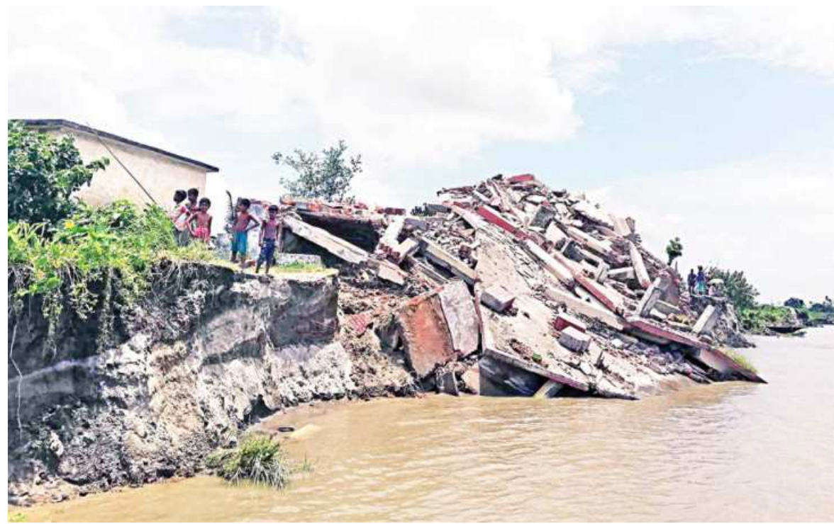
Paiksha Majhail Government Primary School in Tangail lies in ruins after being ravaged by the Jamuna. Many school buildings in the district have suffered a similar fate due to river erosion and ongoing floods. The photo was taken recently.
