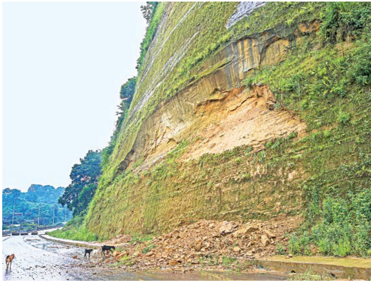
Landslides on multiple parts of the Baizid-Fouzdarhat bypass road in Chattogram -- that was made by cutting hills -- has raised alarm among locals. They said the last few days of rain has caused the small slides, which could be a warning sign for a bigger accident. The photo was taken yesterday.
