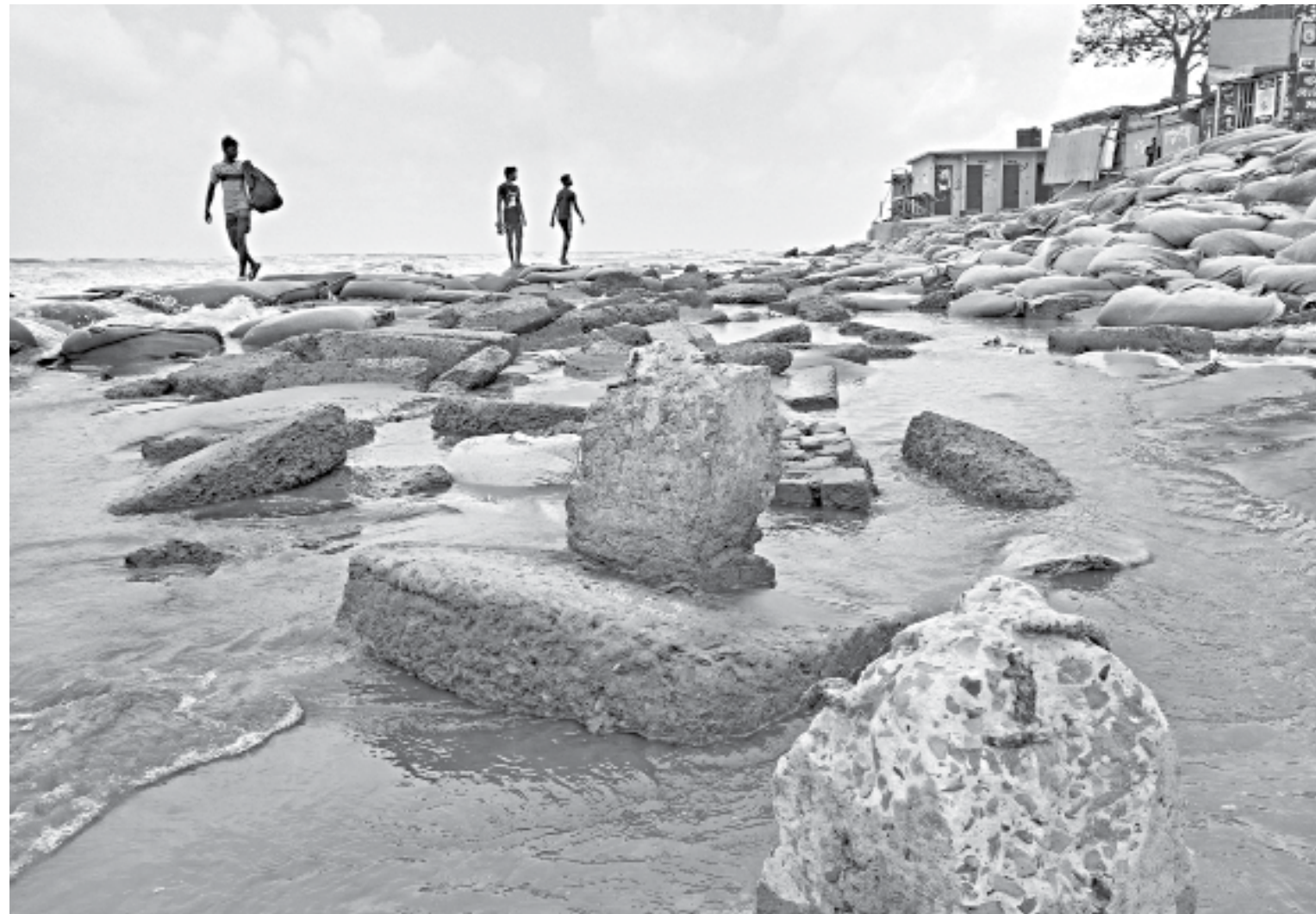
Concrete debris with protruding iron rods and jagged edges scatter the Kuakata beach. The photo was taken on Monday.
