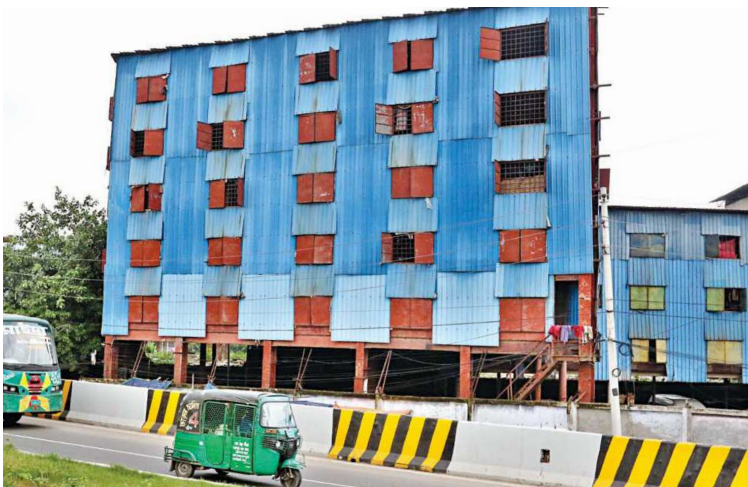
Just across the Postogola Bridge on the outskirts of Dhaka, several of these multistoried residential structures with corrugated metal sheets for walls and a steel platform for a base can be found. While providing presumably affordable housing for mill workers in the area, these do not appear to be safe at all. The photo was taken a few days ago.
