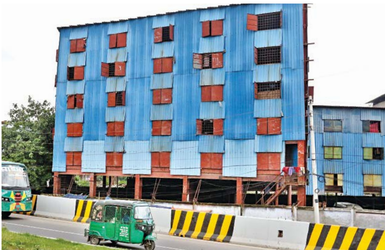
Just across the Postogola Bridge on the outskirts of Dhaka, several of these multistoried residential structures with corrugated metal sheets for walls and a steel platform for a base can be found. While providing presumably affordable housing for mill workers in the area, these do not appear to be safe at all. The photo was taken a few days ago.
