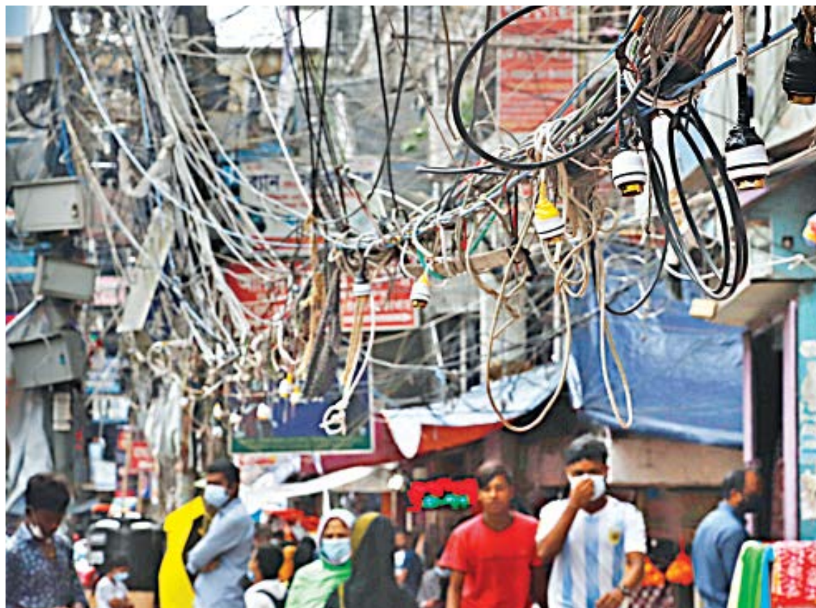
An array of lightbulb sockets hang on a tangle of wires outside the Muktijoddha Super Market in the capital. Roadside hawkers in front of the market use electricity from inside the market by connecting power cables, paying a daily "fare" of Tk 40-50, locals said. Not only is this practice illegal, but the exposed livewire connections on the sockets poses a constant risk of electrocution, especially in rainy weather.
