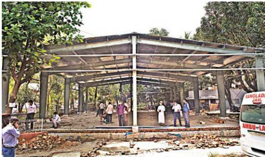
Once completed, this 7,500 sq ft steel structure will help ease long queues and serve additional patients. The photo was taken last week.
