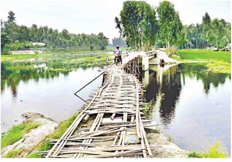
The rush of floodwater washed away the approach road to this bridge in Char Isli village of Rangpur's Gangachara upazila. Desperate for a usable bridge, the locals did not bother to wait for it to be mended. They made it passable by building an approach road out of bamboo poles and fences. The photo was taken yesterday.
