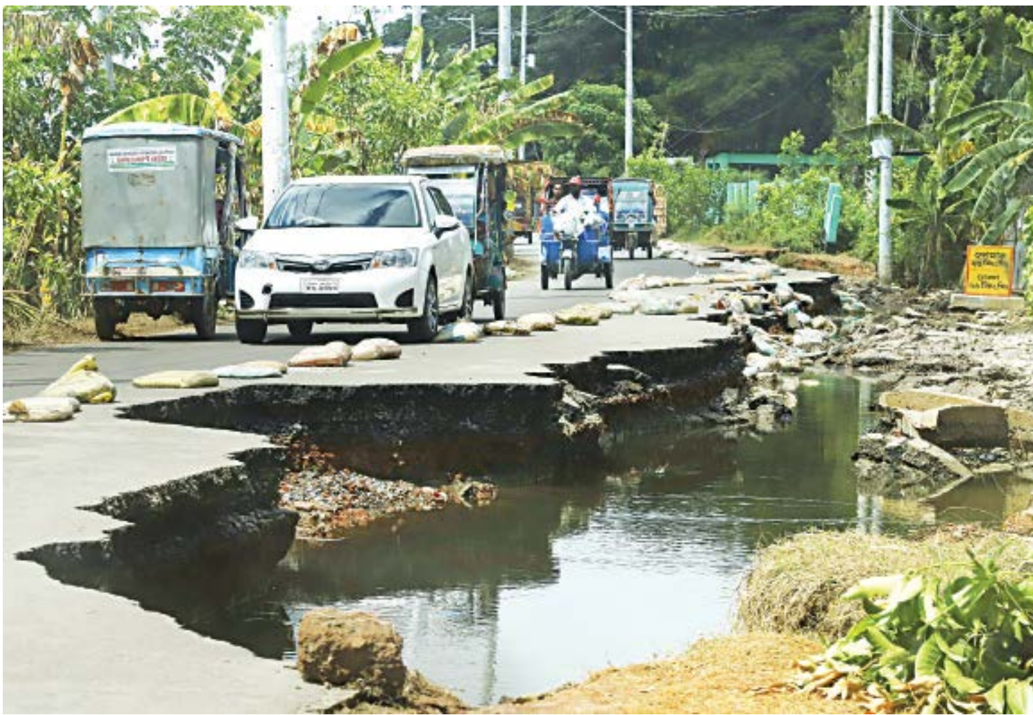
Cars plying Munshiganj's Sreenagar-Dohar road, which is lined with sandbags as it has been heavily damaged due to floods caused by the overflowing of the Padma. Due to enormous cracks, heavy and goods-laden vehicles are not permitted on the road until repair. The photo was taken recently.
