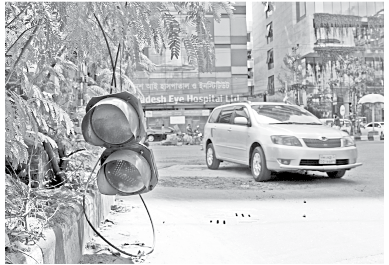
A broken traffic light hangs right in front a pothole on the capital's Dhanmondi Road 27 for weeks, with no one seemingly responsible to fix it. The photo was taken yesterday.
