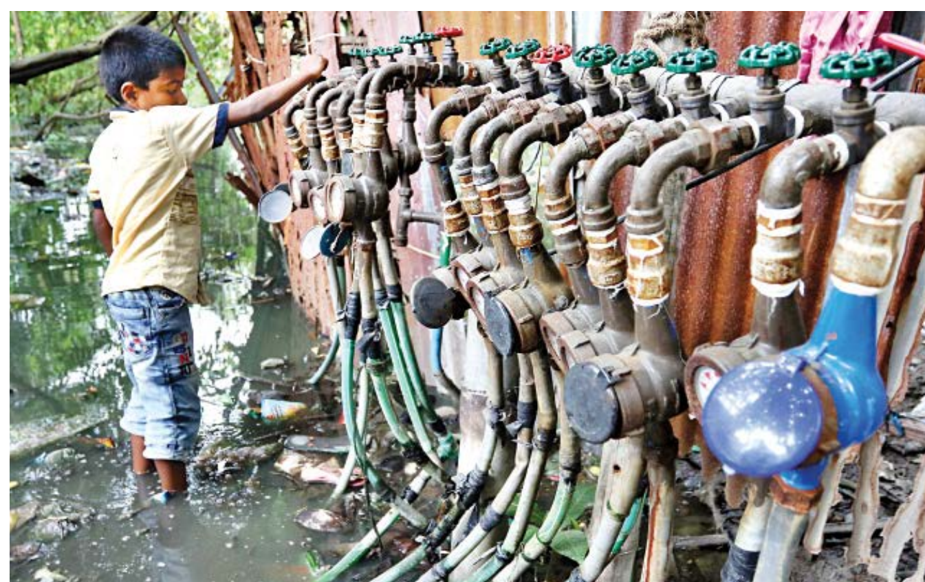
Standing in over ankle-deep water, a boy opens the tap of a line from a water pump in Bagpara of the capital's Nasirabad area. As the locality does not get water supply from Dhaka Wasa, locals have to rely on this pump, which they set up two years ago. Together, they also pay for the electricity needed to pump up the water. Each line supplies water to 70-75 households. The photo was taken on Friday, when the place got waterlogged after rain.
