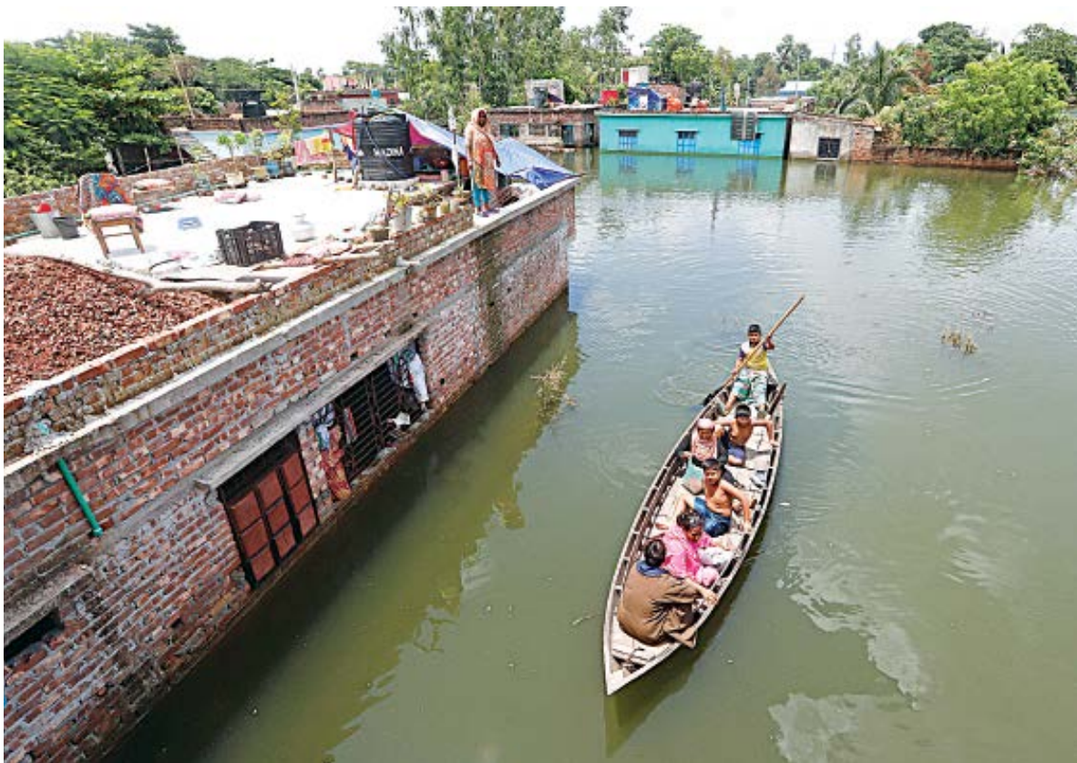
A woman standing on her rooftop watches people on a boat pass by what should be her back yard. Everything downstairs is soaking wet as floodwater ravages the neighbourhood in Makkahnagar area of Savar. Thousands of villages have gone under water and millions have lost everything over the past few weeks. PHOTO: AMRAN HOSSAIN
