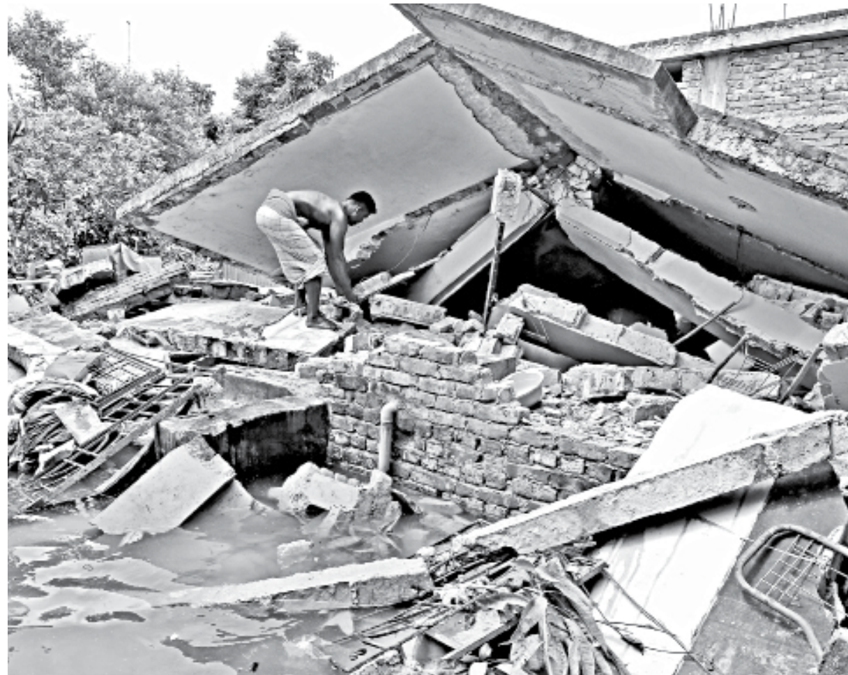
As the flood engulfed roads at Narayanganj's North Narsingpur, this two-storey building collapsed early yesterday. Locals say water gushing into the structure damaged its foundation, and the pillars could not bear the load anymore. Such unfortunate incidents are being reported frequently as over a third of the country has been flooded this year.
