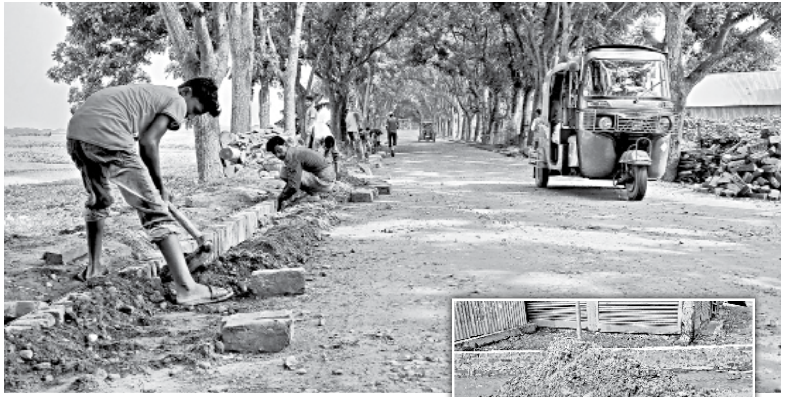
Workers lay bricks along the Akhaura-Chandura road in Brahmanbaria's Bijoy Nagar upazila recently. Inset, a mixture of earth, sand and brick chips of exceedingly low grade is piled up on a side, apparently for using as bitumen macadam surface on the road.
