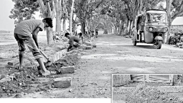
Workers lay bricks along the Akhaura-Chandura road in Brahmanbaria's Bijoynagar upazila recently. Inset, a mixture of earth, sand and brick chips of exceedingly low grade is piled up on a side, apparently for using as bitumen macadam surface on the road. PHOTO STAP
