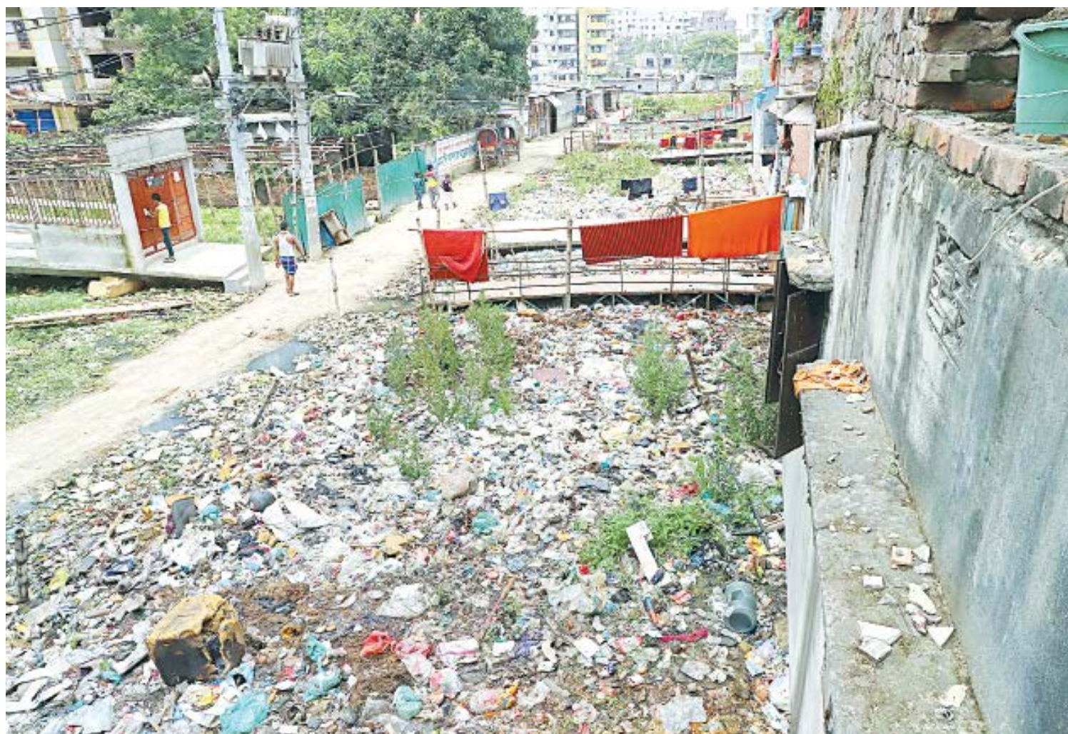
Locals turn Sagunbagicha canal in the capital's North Mughda into a landfill by dumping garbage and plastic items. Such places are ideal breeding grounds for mosquitoes but many are oblivious to the dangers they put themselves and other into by dumping rubbish this way. The photo was taken recently.
