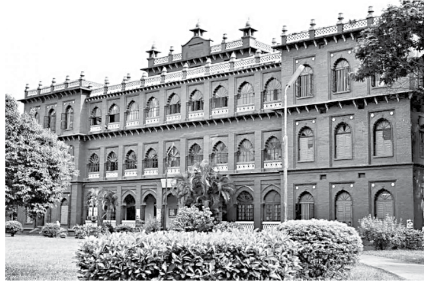
The Curzon Hall building in Dhaka University.
