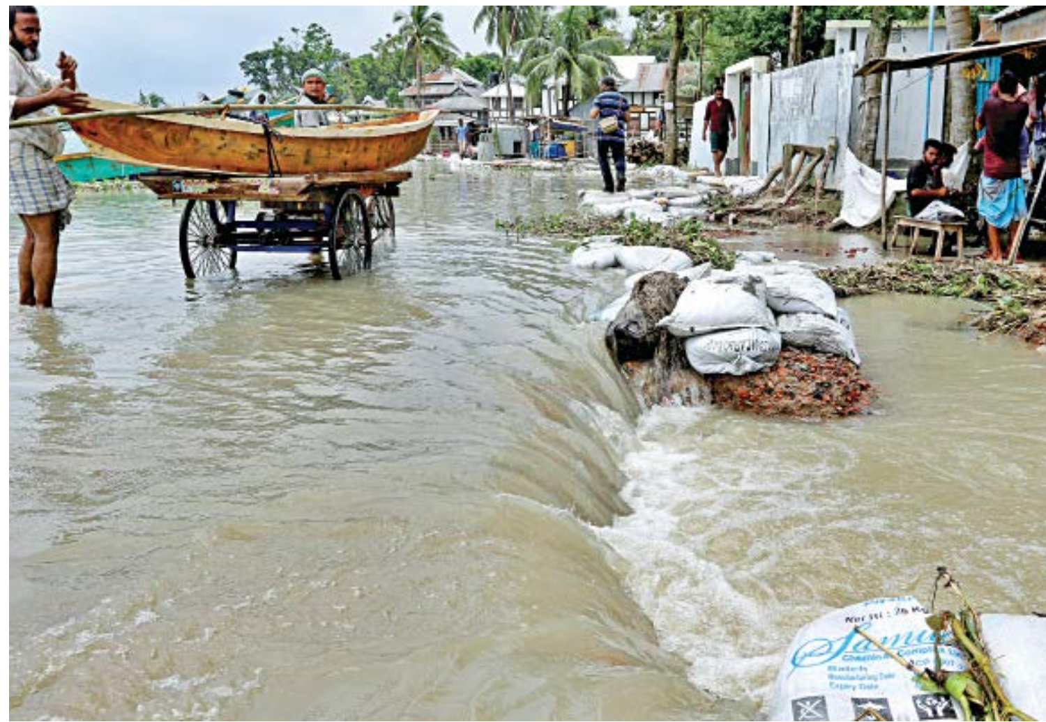
The makeshift dams in Munshiganj's Mawa Kandipara are of little effect against the high current of the overflowing Padma. Floods have beset the country in recent times, and the Padma has swelled beyond danger levels, causing severe damage to houses and roads. This photo was taken on Thursday.
