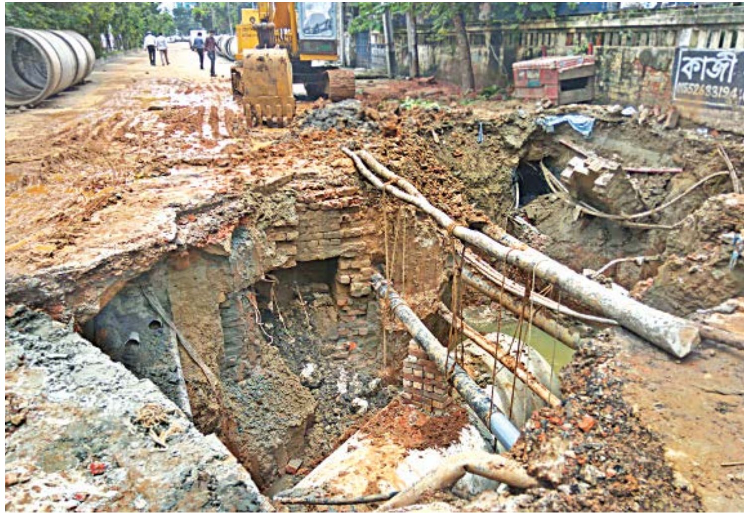
Tying pipes and cables of different utility services to bamboos, Dhaka South City Corporation is installing underground sewerage pipes to widen the lines at Dhanmondi-27. Locals allege that they are suffering immensely as the work progresses slowly. Rainwater also adds to their woes. The photo was taken yesterday.
