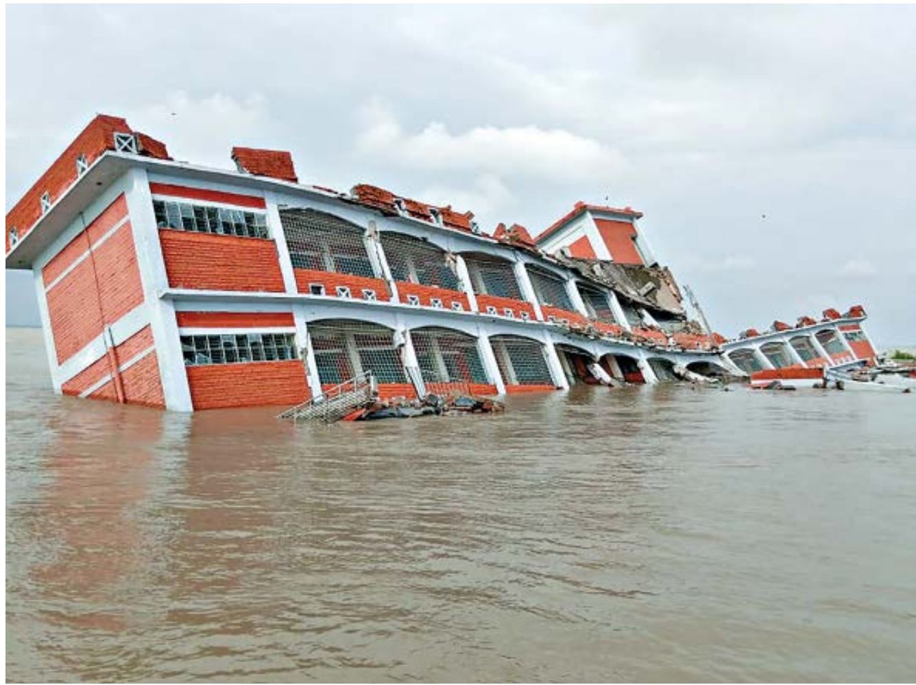
The three-storey building of Nuruddin Matborerandi Model High School is warped out of shape as the ground on which it stood is being washed away by the Padma. The building was barely visible soon after the photo was taken around 5:30pm yesterday in Bandarkhola union of Madaripur's Shibchar upazila. When schools reopen, students of at least 24 villages will have to travel to schools far away from their homes.
