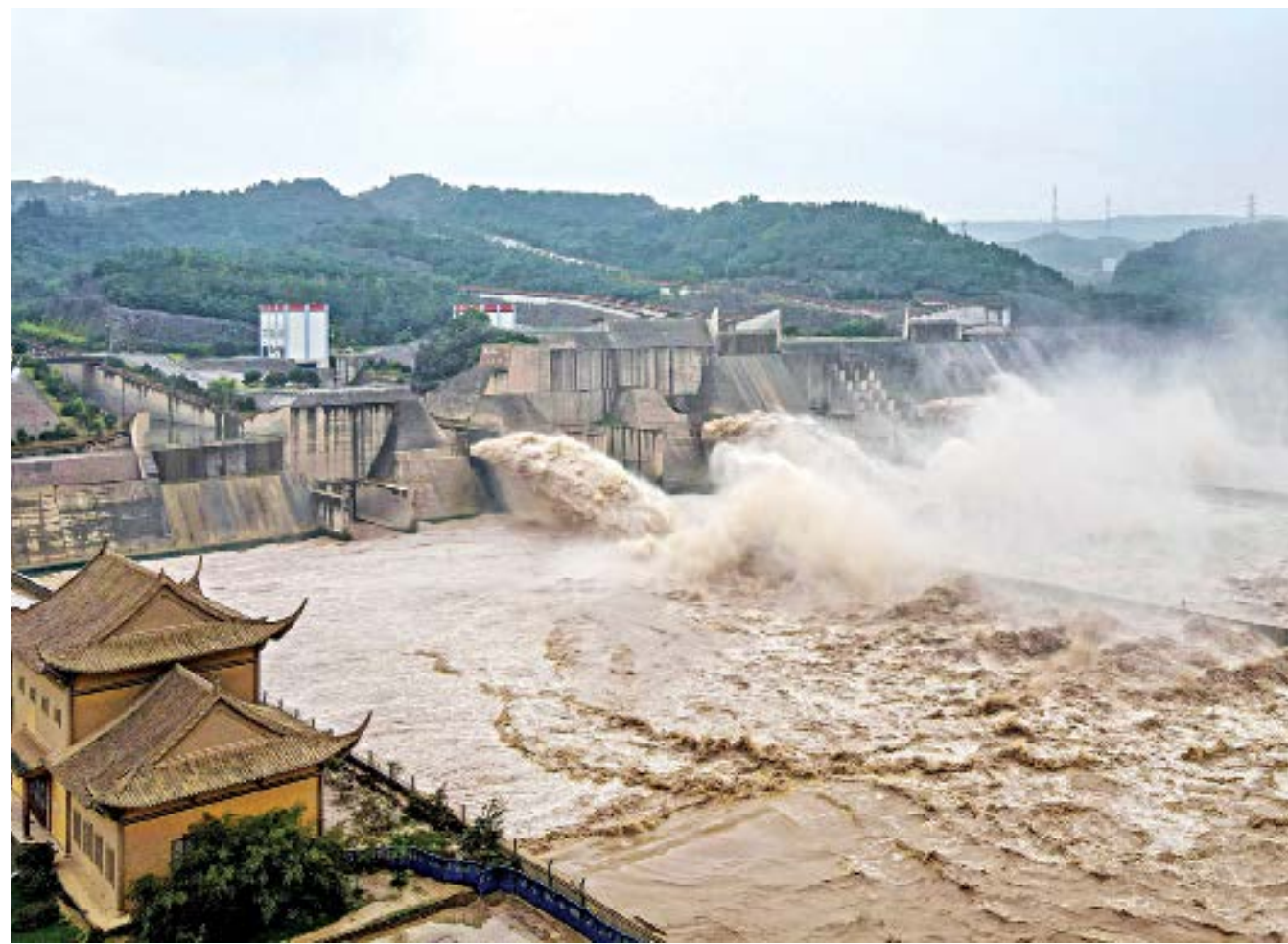
This aerial photo taken on Sunday shows water released from the Xiaolangdi Reservoir Dam in Luoyang in China's central Henan province, in preparation of the upcoming annual flood season at the Yellow River basin.
