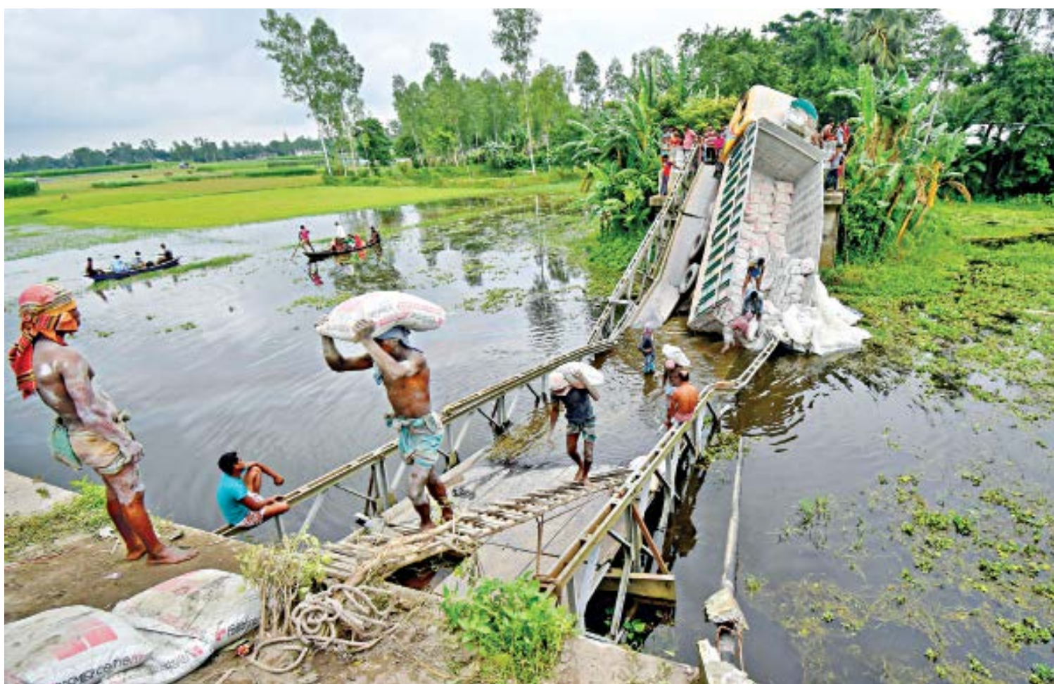
Workers salvage cement bags from a lake and people go across it by boats after the narrow bailey bridge, with a load-bearing capacity of 15 tonnes, collapsed while a truck carrying around 47 tonnes of cement bags drove over it yesterday morning, officials said. The bridge on Barungi Beel in Bogura's Gabtali upazila linked the flood-hit Sariakandi upazila with the rest of the district. Engineers said they will sue the truck owner and its driver. Over a couple of lakh people will suffer until a new truss bridge is constructed and open to traffic in about a week.
