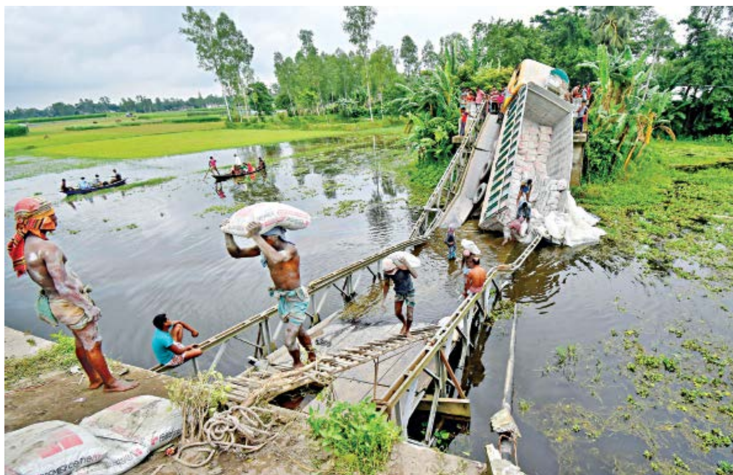
Workers salvage cement bags from a lake and people go across it by boats after the narrow bailey bridge, with a load-bearing capacity of 15 tonnes, collapsed while a truck carrying around 47 tonnes of cement bags drove over it yesterday morning, officials said. The bridge on Barungi Beel in Bogura's Gabtali upazila linked the flood-hit Sariakandi upazila with the rest of the district. Engineers said they will sue the truck owner and its driver. Over a couple of lakh people will suffer until a new truss bridge is constructed and open to traffic in about a week.
