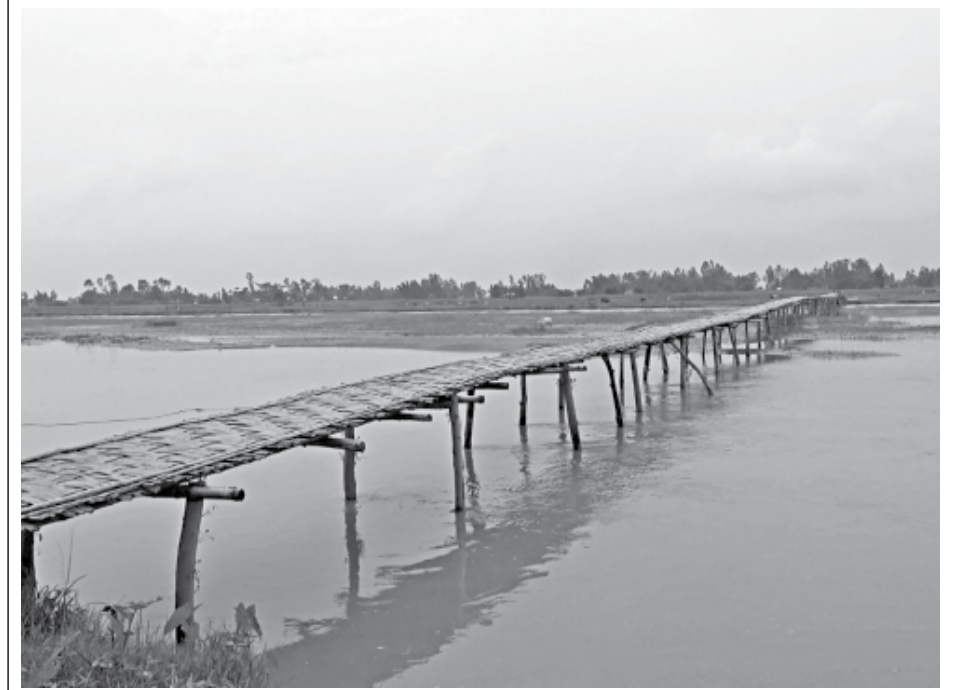
Char people in Khuniyagachh union of Lalmonirhat Sadar upazila build the bamboo bridge on a canal of the Teesta river on self-help basis to ease their communication.
