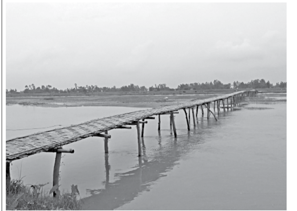
Char people in Khuniyagachh union of Lalmonirhat Sadar upazila build the bamboo bridge on a canal of the Teesta river on self-help basis to ease their communication.
