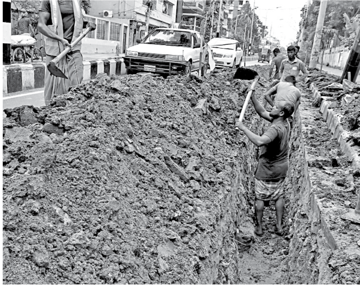
Dhaka Electric Supply Company (Desco) has chosen an inopportune time to dig up this road in Mirpur-1 for work on underground cable lines, as rainy weather may not just slow the work down but also pose hassles to commuters. Locals said the road was renovated just a year ago and was in perfectly good shape until the excavation. The photo was taken yesterday.
