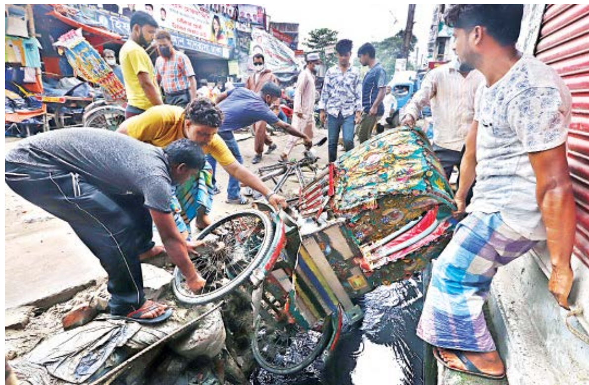
Passersby on Zia Sarani in the capital's Shanir Akhra help a rickshaw-puller retrieve his vehicle after it fell into Kutubkhali canal. A portion of the culvert over the canal collapsed about eight months ago, narrowing it to such an extent that two vehicles can hardly pass at a time. The photo was taken yesterday.
