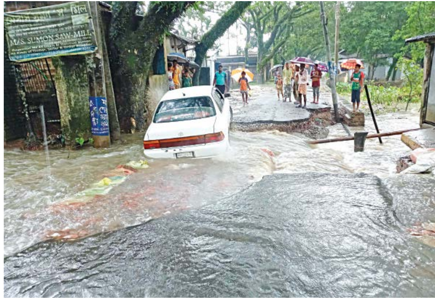
A car struggles to get off a damaged portion of an inundated road in Sunamganj town's Nabinagar area yesterday. A part of the road caved in due to strong currents of water from the Surma river, which has started flowing above the danger level since Thursday afternoon. Some low-lying areas of the town are going under water, causing floods.
