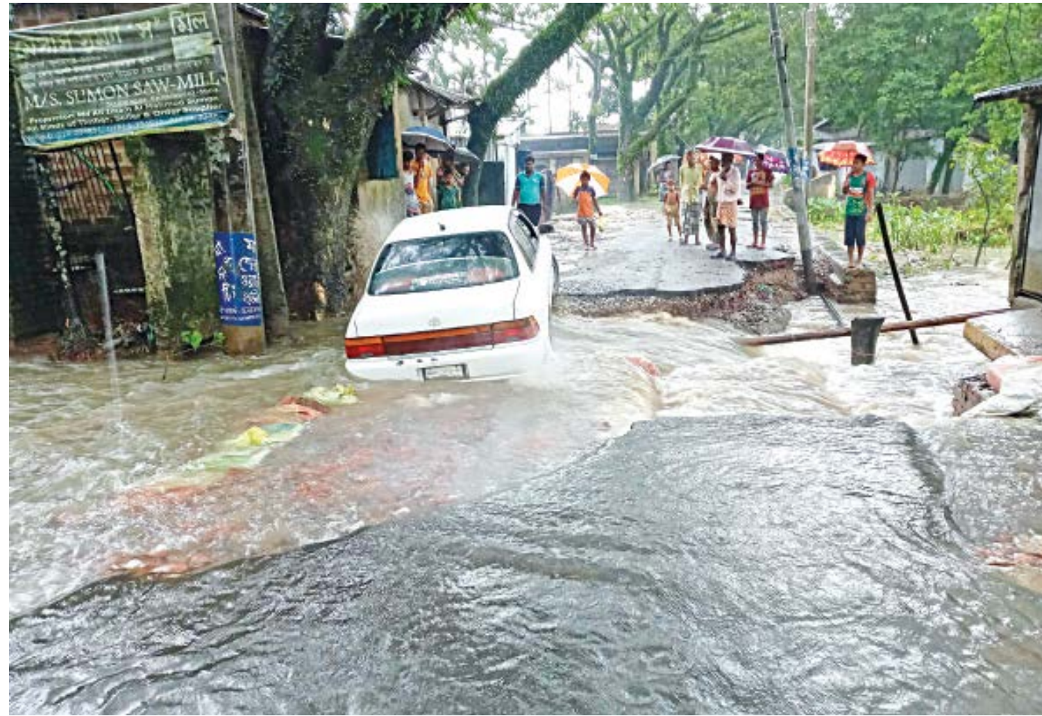
A car struggles to get off a damaged portion of an inundated road in Sunamganj town's Nabinagar area yesterday. A part of the road caved in due to strong currents of water from the Surma river, which has started flowing above the danger level since Thursday afternoon. Some low-lying areas of the town are going under water, causing floods.
