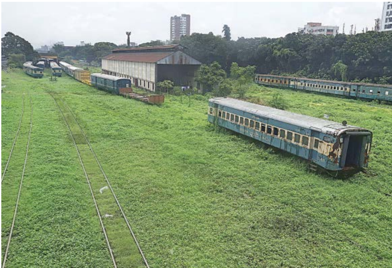
A lush vegetation appears to be reclaiming the stabling area at Kamalapur rail station in the capital. With a fraction of the fleet of trains operating after over two months of shutdown, the pre-pandemic hustle and bustle has yet to return to the terminal. The photo was taken yesterday.
