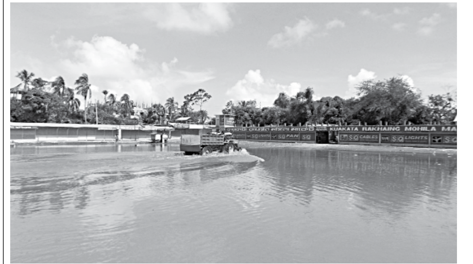
Kuakata Rakhine Mahila market's field in Patuakhali's Kalapara upazila remains inundated for six months of the year due to lack of proper drainage system.
