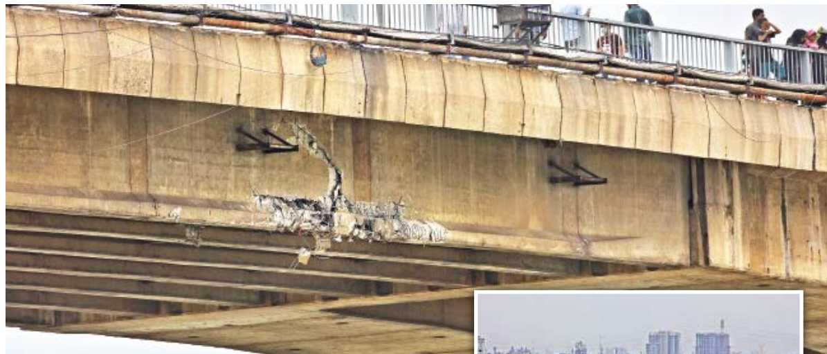
The damaged portion of the Postogola bridge on the Buriganga. The crane, inset, of BIWTA rescue ship Prottoy hit the structure on Monday while going to salvage the sunken launch Morning Bird in Sadarghat area. Movement of traffic on the bridge remained suspended since Monday evening. The photos were taken yesterday.
