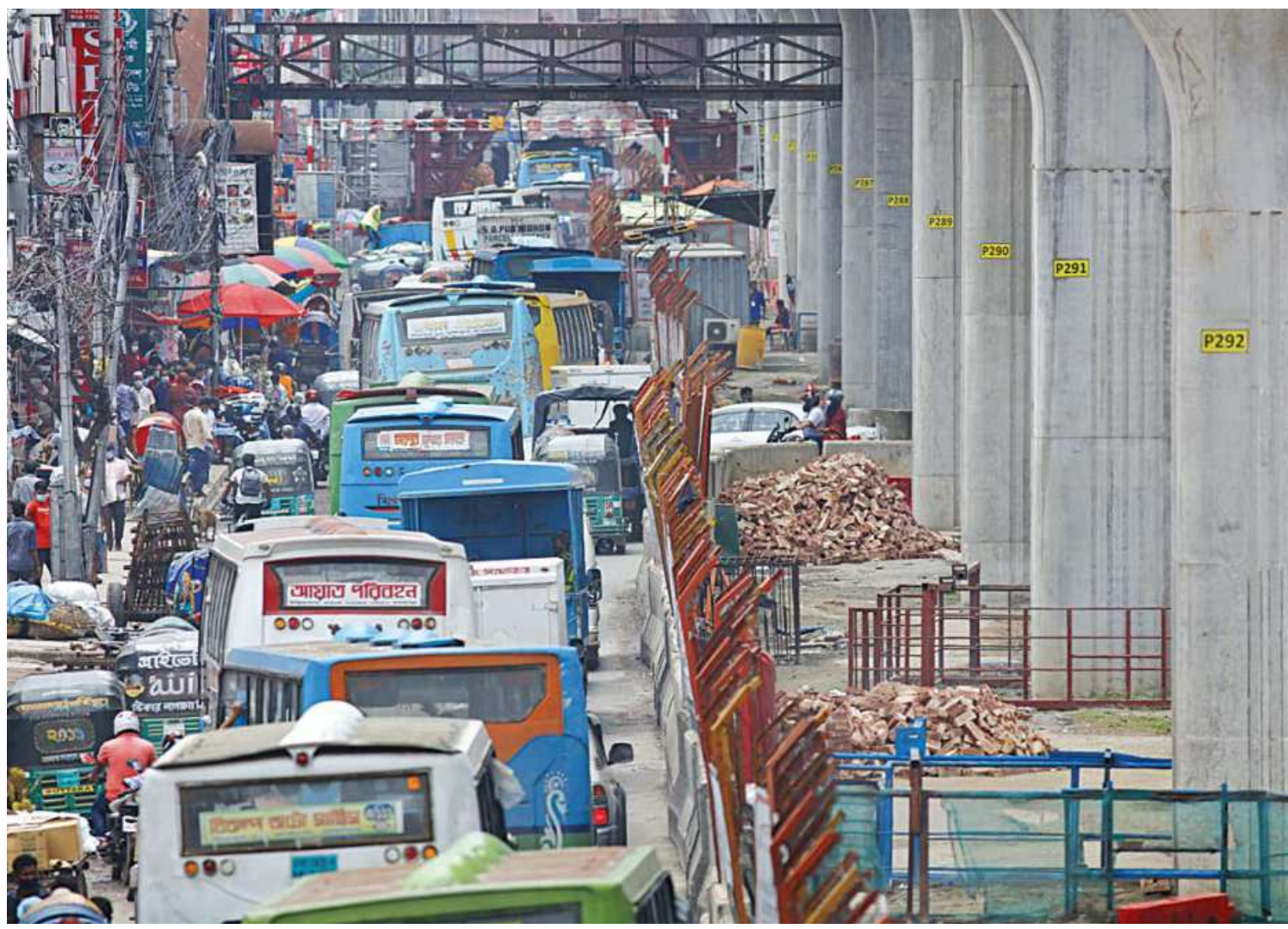
Vehicles clog the Rokeya Sarani in the capital yesterday as metro rail construction work resulted in almost halving of the road width there.
