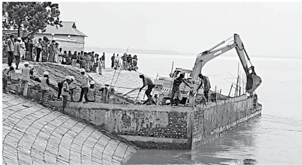
Workers engaged by Kalihati upazila administration dismantling a permanent structure constructed illegally on a village protection embankment along the Jamuna in Gorilabari village of the upazila.
