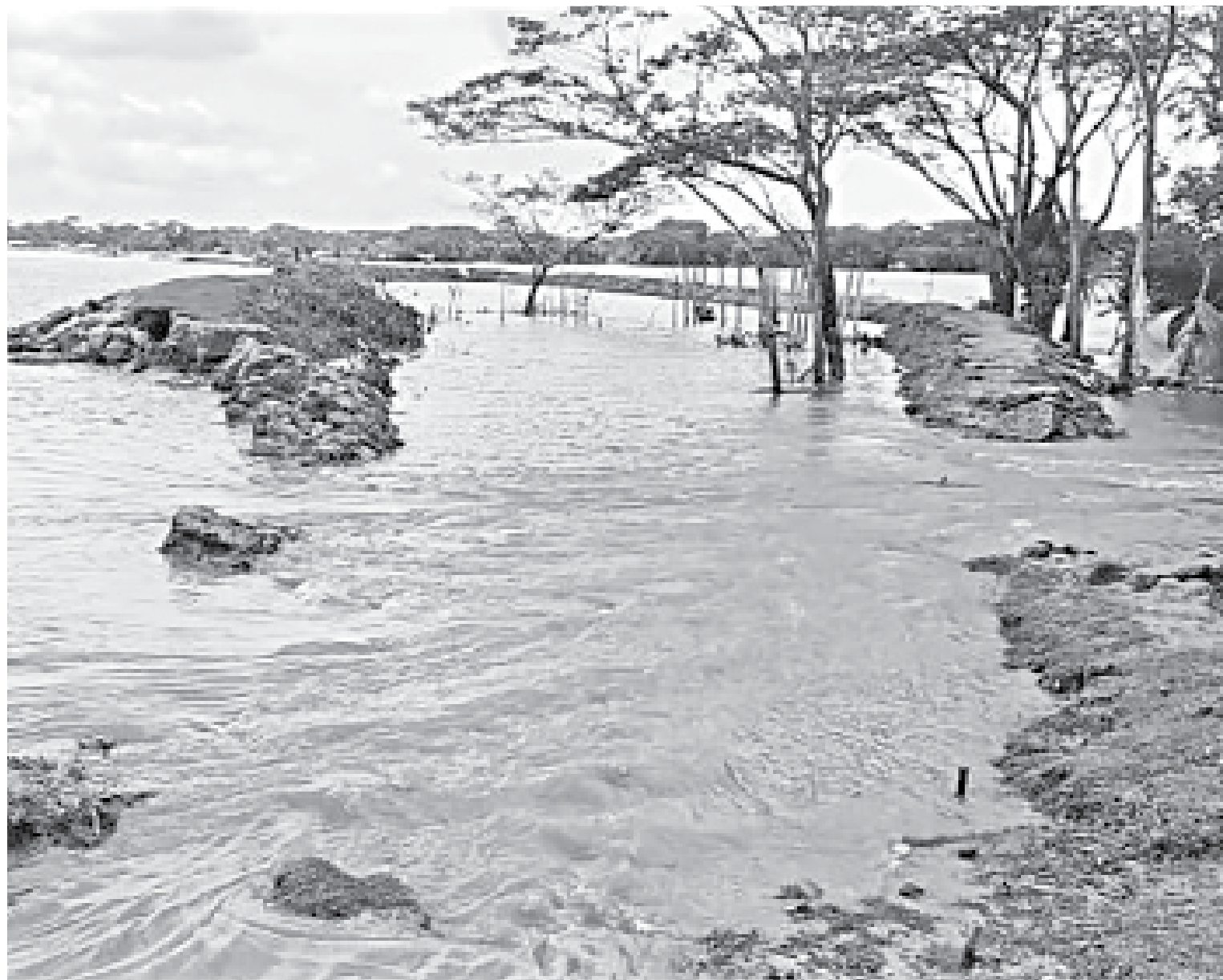
Water rushing through the breached portion of this embankment at Bogigabola village in Bagerhat's Sharankhola upazila has flooded the locality, adding to the woes of the people who are still reeling from the destruction caused during the onslaught of super cyclone Amphan on May 20.
