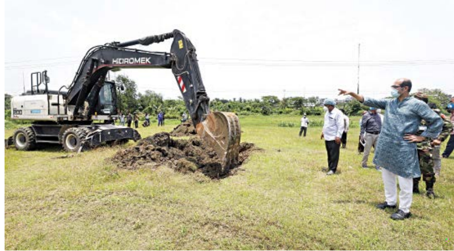
Mayor Atiqul Islam oversees canal excavation works yesterday. PHOTO: COLLECTED
