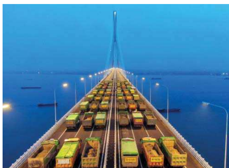
This aerial photo taken on Wednesday shows trucks driving on the Hutong Yangtze River Bridge during a load test in Nantong, in China's eastern Jiangsu province.
