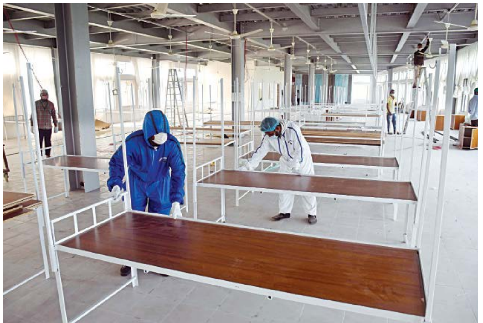
A 120-bed quarantine centre being readied by AL Muslim Group at its factory in Ulail area of Savar on the outskirts of the capital. The apparel manufacturer will keep any of its workers, suspected to have contracted the novel coronavirus, at this facility. The photo was taken on Sunday.
