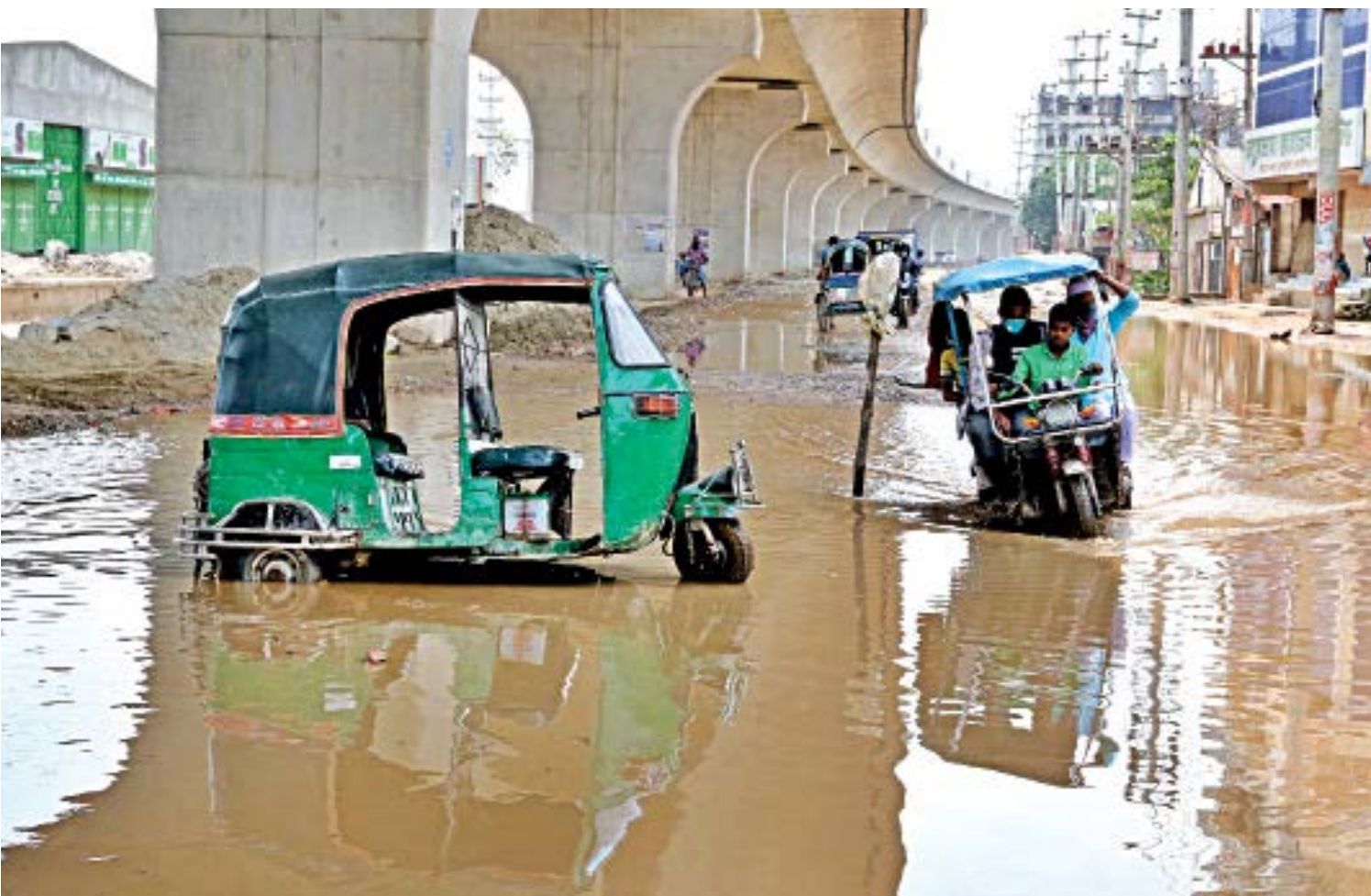
After the downpour of the past few days, the road beneath Jinjira overpass (that goes from Dhaka to Mawa) has been severely damaged and waterlogged. While larger vehicles like trucks can still pass through, CNG-run autorickshaws and smaller vehicles are getting stuck in the muddy street that runs for almost a kilometre. The photo was taken yesterday.
