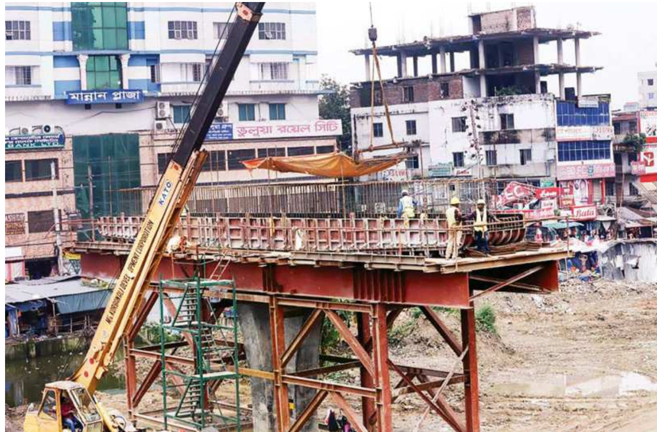
Construction of the elevated expressway in progress at Airport Road.
