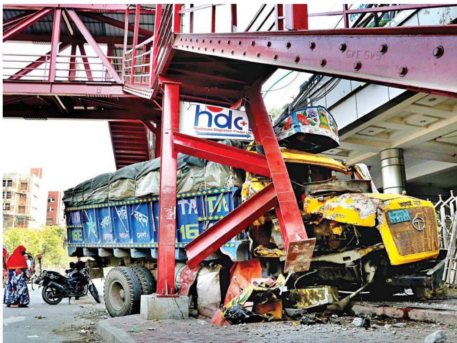
A goods-laden truck lost control and crashed into a newly-built footbridge in Shyamoli on Mirpur Road early yesterday, severely damaging the structure. Had the roads not been empty due to the coronavirus outbreak, the damage could have been much more serious.
