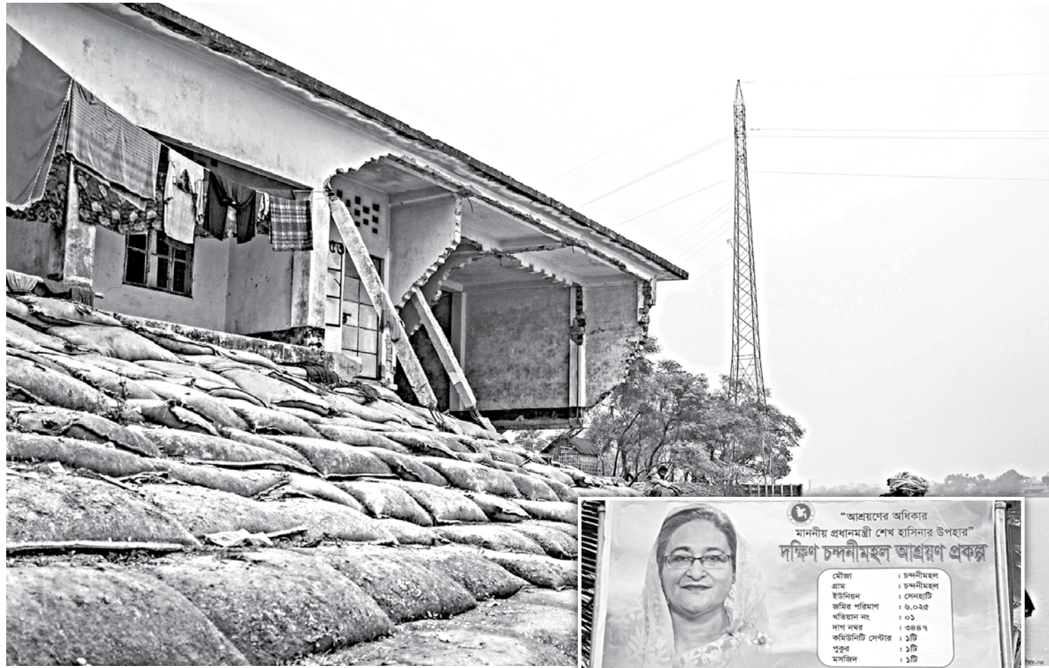
Geotextile sand bags were dumped on the Atai river bank where a barrack of 'Dokkhin Chandonimahal Ashrayan Prokolpo', Inset , a government housing project for the landless in Digholia upazila of Khulna, was damaged due to erosion.
