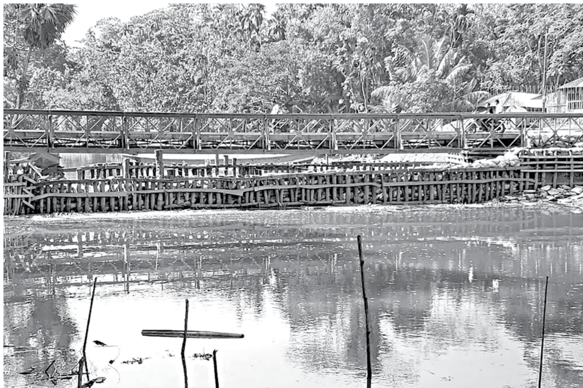
A group of local people build an illegal dam in Varani Khal of Barishal's Bakerganj upazila to stop erosion by river.
