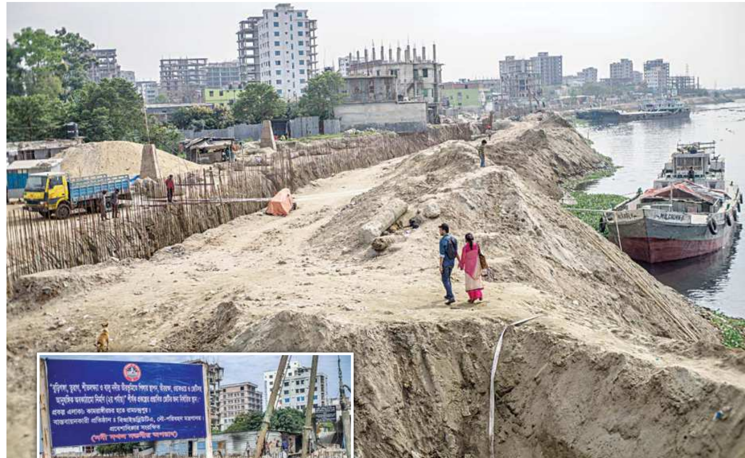
A part of the Buriganga river earth-filled by the Bangladesh Inland Water Transport Authority in Ramchandrapur area of Mohammadpur in the capital. The irony is that BIWTA's signboard, inset, in the area says river grabbing is a punishable offence. The photo was taken yesterday.
