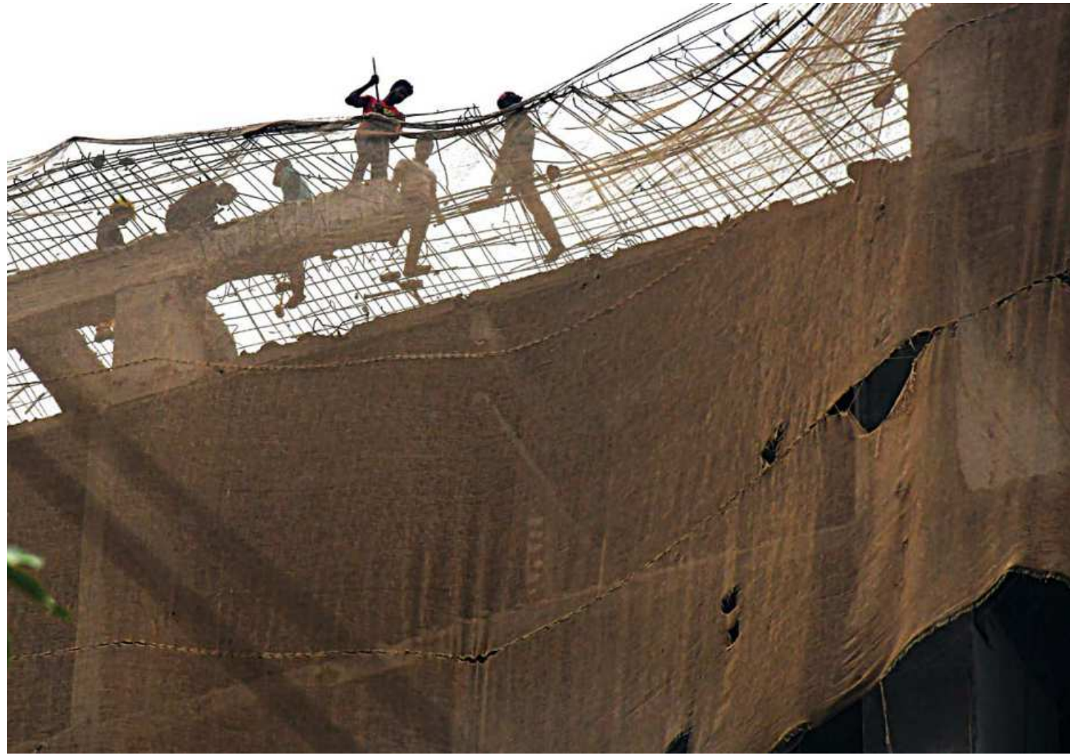
With no safety gears on, workers knocking down the BGMEA Bhaban, illegally built on Hatirjheel, in the capital's Karwan Bazar area yesterday. Their disregard for safety puts them at risk.
