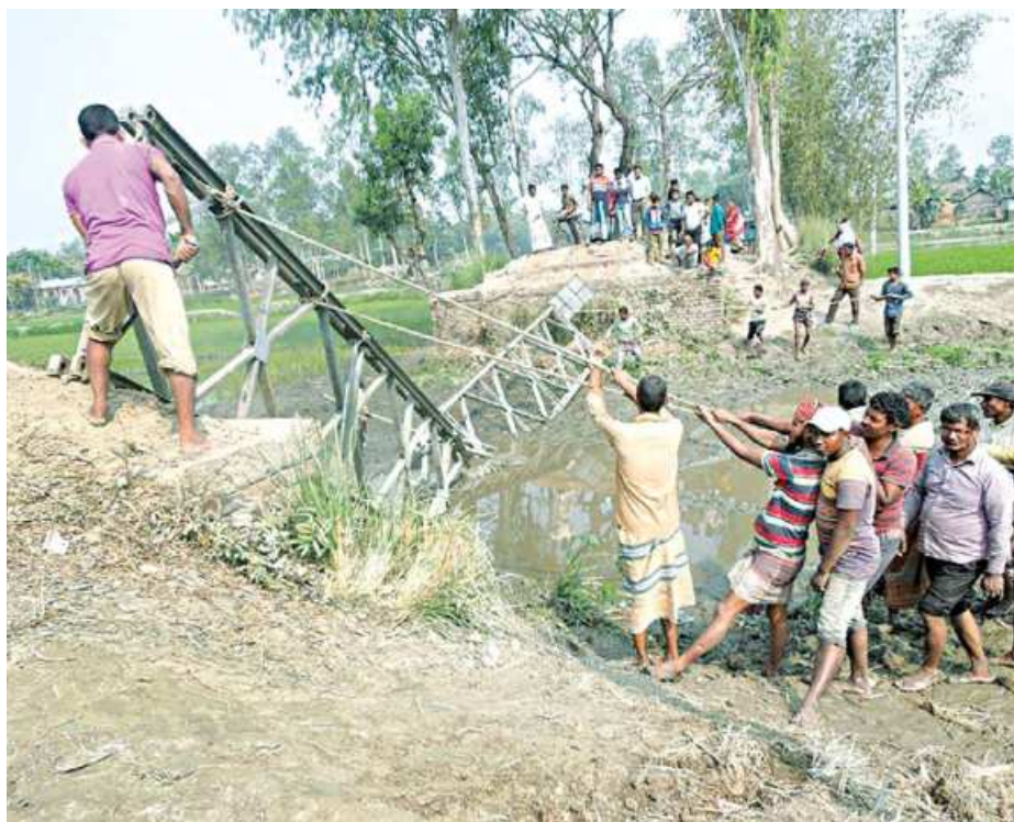
Road communication between Nilphamari Sadar and Chilahati land port has remained suspended since Thursday night after a Bailey bridge near Banunia area in Domar upazila collapsed when an overloaded cement-carrying truck was crossing it. Ignoring warning from the authorities concerned, heavy vehicles had continued using the bridge.
