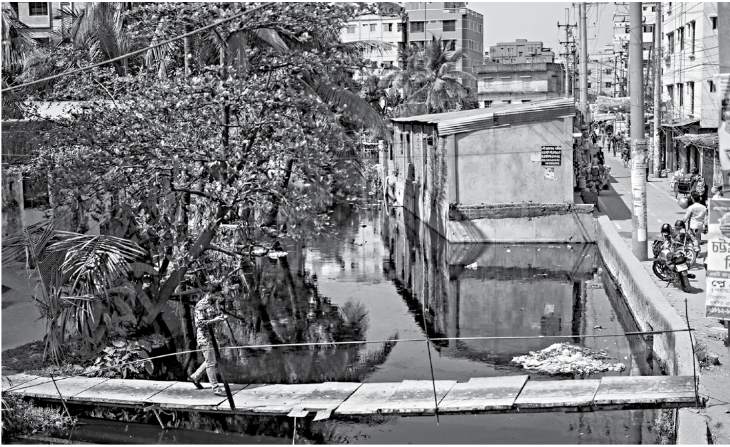
A tin-shed structure has been constructed on Chattogram's Chaktai canal. Transgressions into waterbodies like this have become a regular occurrence across the country. This photo was taken yesterday.
